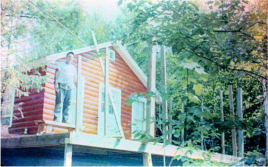
Addition being built following the first summer
