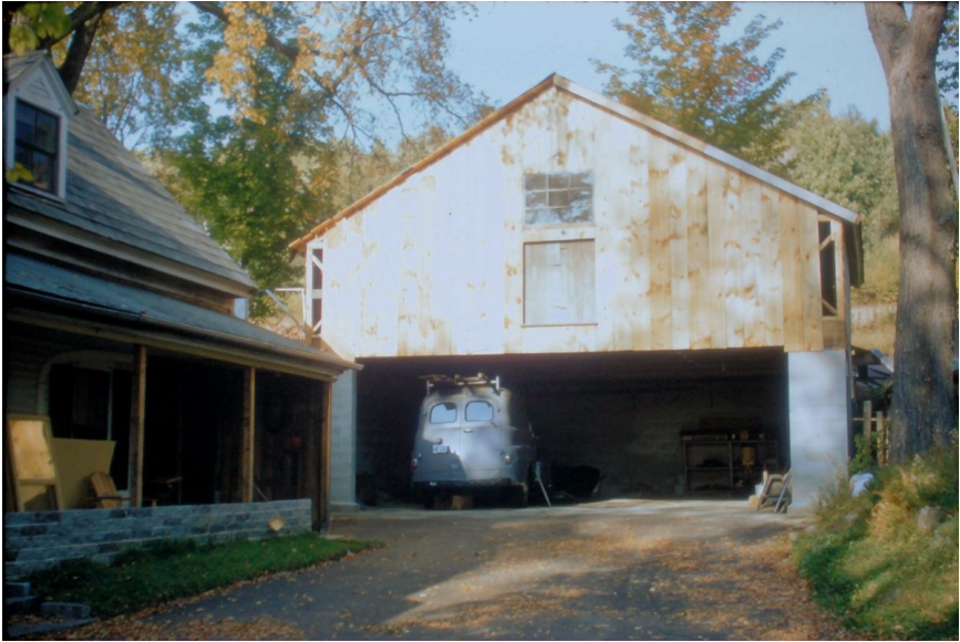
Newly built garage - 1955
